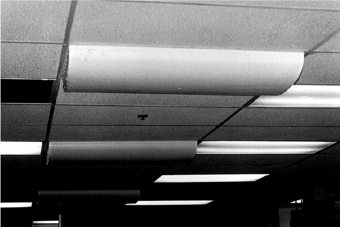
*Figure 4: Supply Diffuser Replacements*
