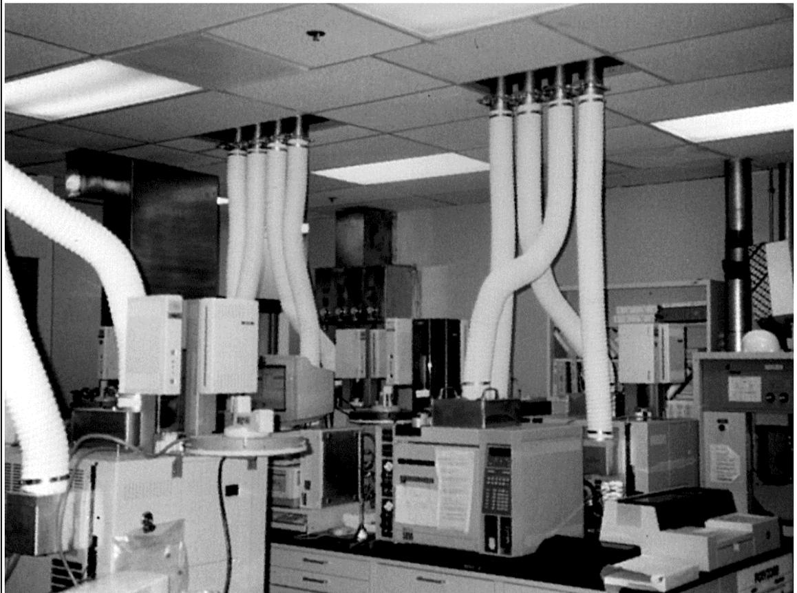
Figure 6: Gas Chromatograph Ventilation System
